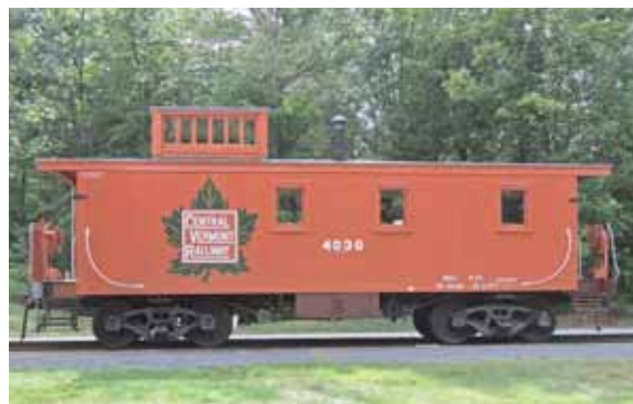
The Central Vermont Railway caboose in Potter Place in September 2022, after the stencils and herald have been applied. Some painting of the exterior remains to be finished.
