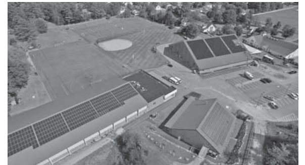
Proctor Academy completed the installation of its 11th solar array this summer, a one acre, 412,000 kwh array on the Farrell Field House.
