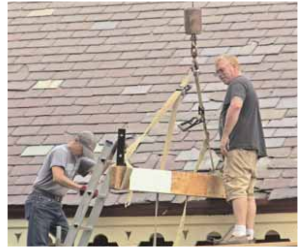
In other Potter Place news, Fred Nystrom and Doug Colby, volunteers for the Andover Historical Society, install the horizontal "Train Order Signal" (semaphore) support beam.
